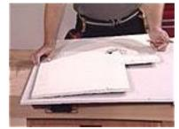
If the damaged area came out in one piece, use that section as a template when cutting a patch. Be sure to match the tapered area of the new piece with that of the old one.
