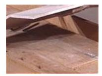
Score the drywall's paper with a knife, then simply snap the area to be cut out.
